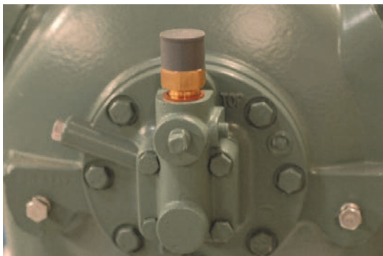
Fig. 23 — OPSS Sensor Installed
