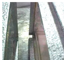
Blower Section (left) and bottom of coil (right) with \frac{3}{4} " slot.
