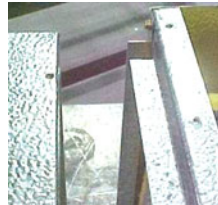
Blower Section (left) and top of coil (right) with \frac{3}{4} " slot.
