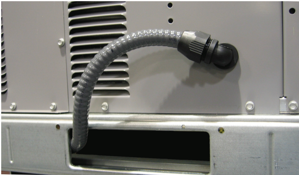
Fig. 4 - Detail showing drip loop to prevent water from collecting in liquid tight conduit.
