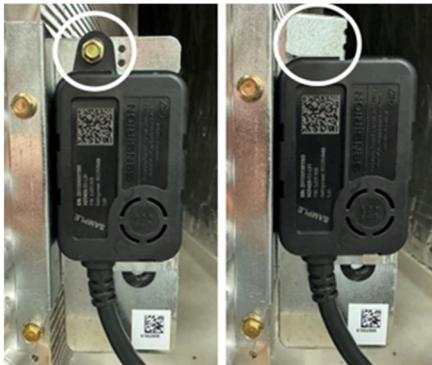
3. Secure the sensor cable using the provided cable clamp and screw in the general area shown below. Ensure a drip loop is created per the previous instructions. Take care to ensure the screw does not pierce the evaporator coil.
