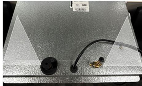
2. Locate the knockout on the coil panel and remove it. Install the split grommet and route the sensor cable through the panel.
