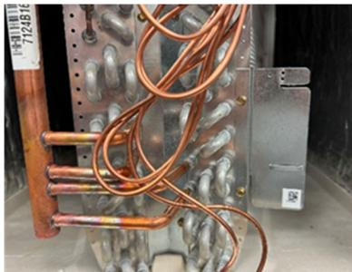
1. Insert the sensor into the slot with the cable routed downwards then bend the top tab or install the provided screw as shown below, to lock the sensor in place.
