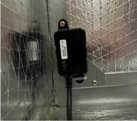
2. Locate the knockout on the coil panel and remove it. Install the split grommet and route the sensor cable through the panel.
