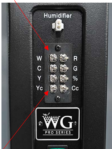
24-volt, two-position terminal block
