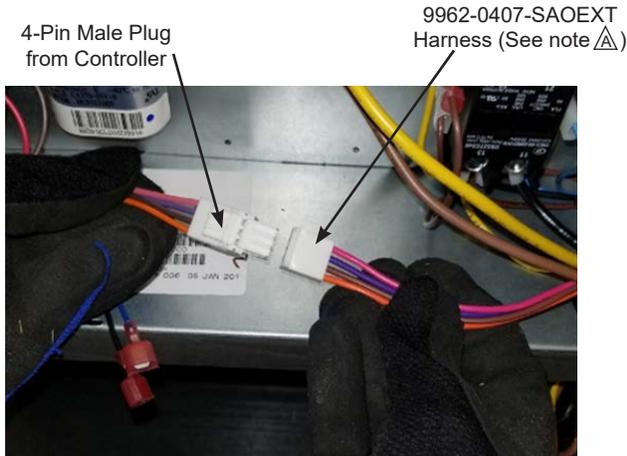
**Figure 13 – Connect 9962-0407-SAOEXT Harness to Harness from Controller (See note below)**
