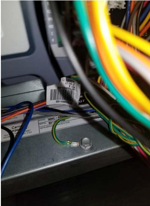
**Figure 12 – Connect Ground Wire From Controller**
