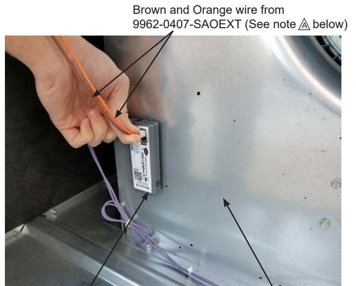
**Figure 15 – Mount and connect Mixed Air Sensor**
