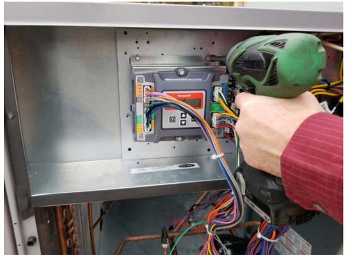
**Figure 7 – Mount Controller Assembly in Unit Control Box**
