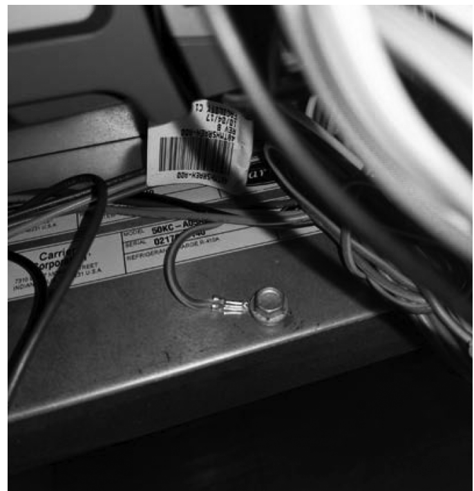
Fig. 13 — Connect Ground Wire From Controller
