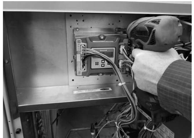
Fig. 8 — Mount Controller Assembly in Unit Control Box
