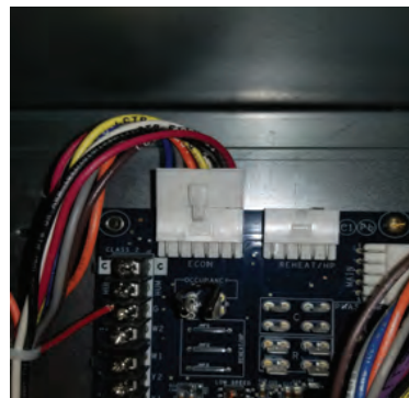
Fig. 12 - Connect 12-Pin Plug to Unit Control Board
