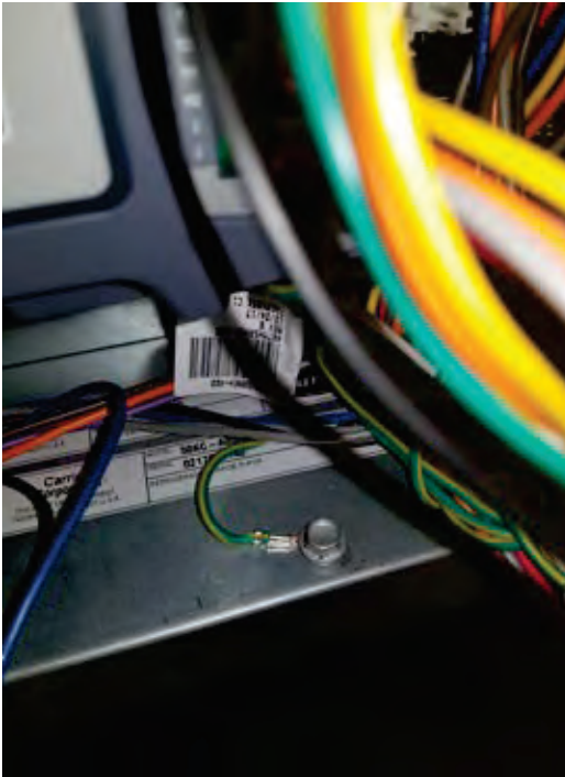
Figure 20 – Connect Ground Wire From Controller
