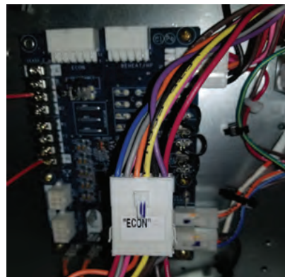
Fig. 11 — Connect 12-pin Plugs Together
