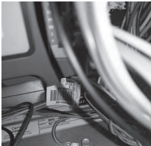
Fig. 13 — Connect Ground Wire From Controller
