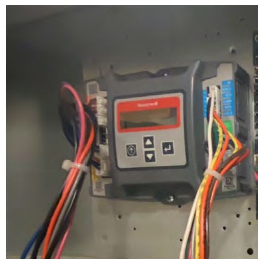
Figure 7 – Mount Controller Assembly in Unit Control Box
