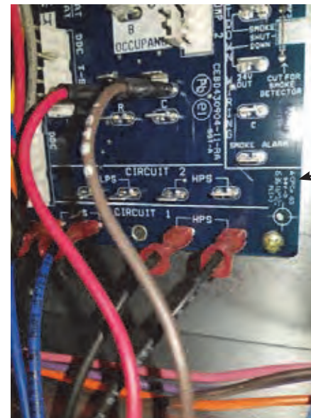
Figure 19 – Connect Red and Brown Wires to Central Terminal Board
