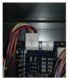
Fig. 14 — Connect 12-Pin Plug to Unit Control Board
