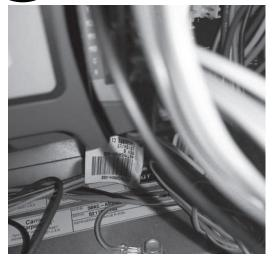
Fig. 15 — Connect Ground Wire From Controller
