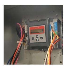
Figure 11 – Mount Controller Assembly in Unit Control Box
