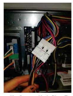
Figure 19 - Connect 10-pin Plugs Together
