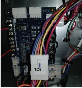
Fig. 13 — Connect 12-pin Plugs Together
