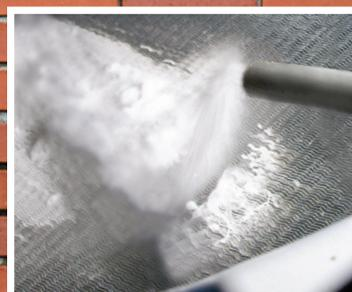
Foaming action lifts and cleans dirt and debris.
