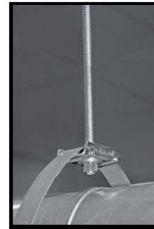
Spiral Buckle with threaded rod
