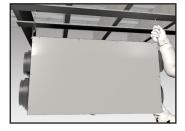
3 Hang the unit by slipping a link onto the hanging hooks, making sure the unit is level.
