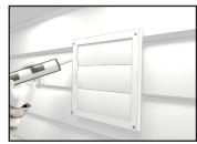
**4** Using a caulking gun, seal around both hoods to prevent any leaks.
