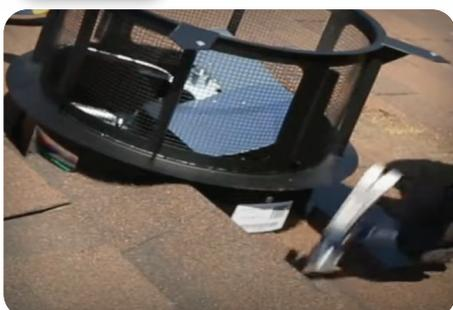
10. Apply weatherproof sealant all around the fan housing and secondary flashing, closing the gap between the flashing, the fan unit, and the tile. Using an angle grinder, cut the removed tiles as needed. Re-install the tile around the fan unit.
