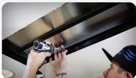
8. Using the included drywall screws, fasten the damper box to both the drywall and the joist in the attic.
