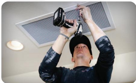
9. Remove ceiling grille and screws from its packaging. Center the grille over the damper box. Install the grille with the white screws provided by screwing through the drywall into the flange of the damper box.
