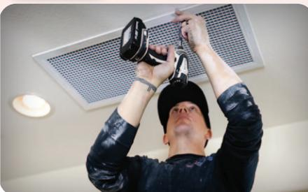
9. Remove ceiling grille and screws from its packaging. Center the grille over the damper box. Install the grille with the white screws provided by screwing through the drywall into the flange of the damper box.
